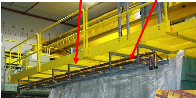
Platform water manifolds and cable trays
