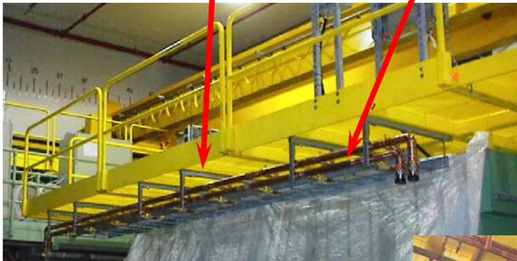
Platform water manifolds and cable trays
