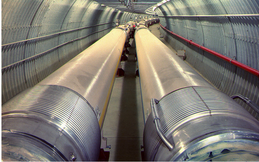
Figure 2.2: Photograph inside the RHIC tunnel showing the two concentric rings of beam tubes [47].
